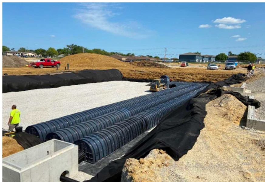
Figure 1 - Typical HydroChain™ Chamber Storage System
