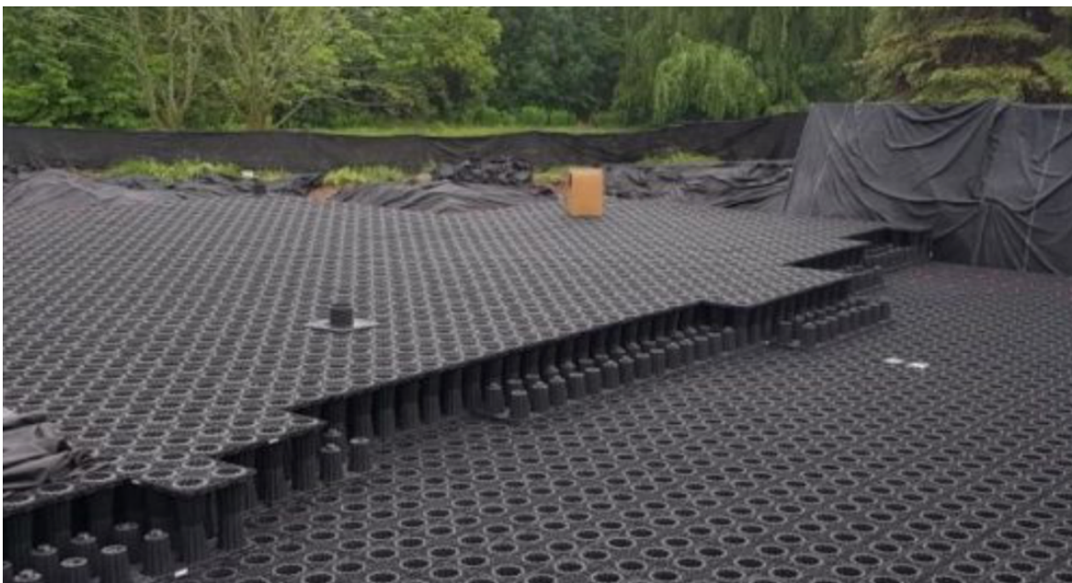
Figure 1 - Typical StormBrixx System
